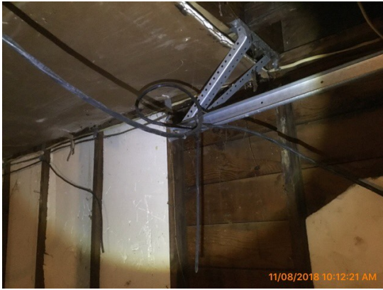
West garage at overhead door rail
