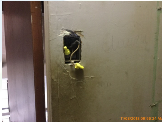
Upstairs closet north
