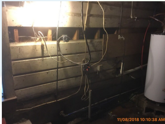
East garage wall
