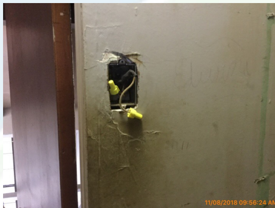
Upstairs closet north
