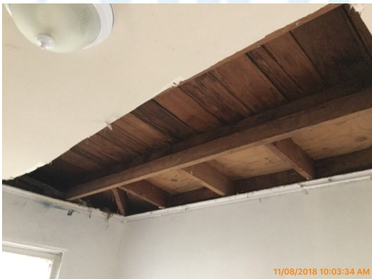
Upstairs southwest bedroom
