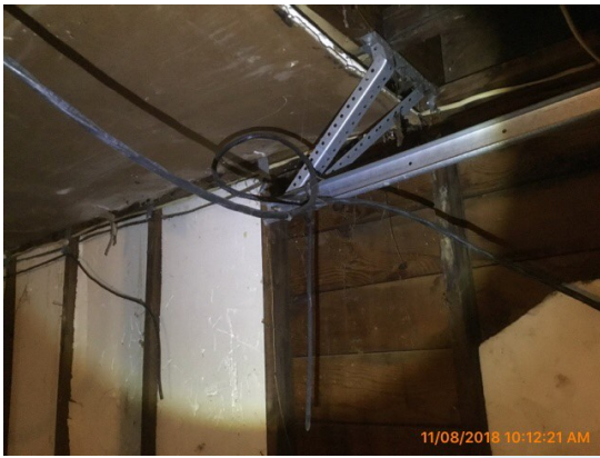
West garage at overhead door rail
