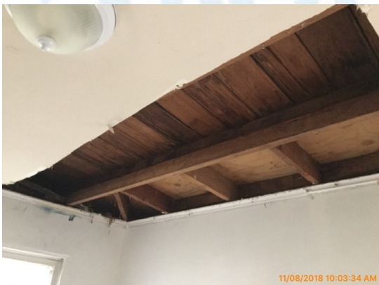
Upstairs southwest bedroom
