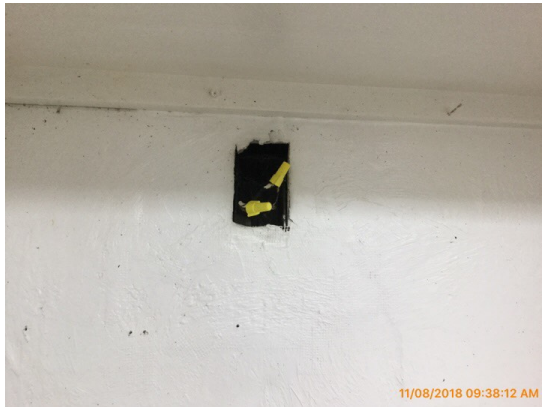
South wall kitchen at refrigerator cavity.
