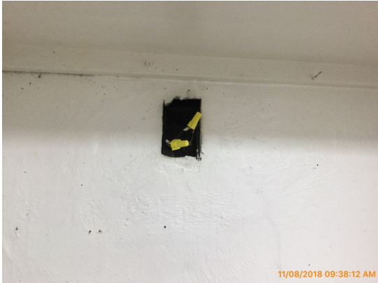
South wall kitchen at refrigerator cavity.
