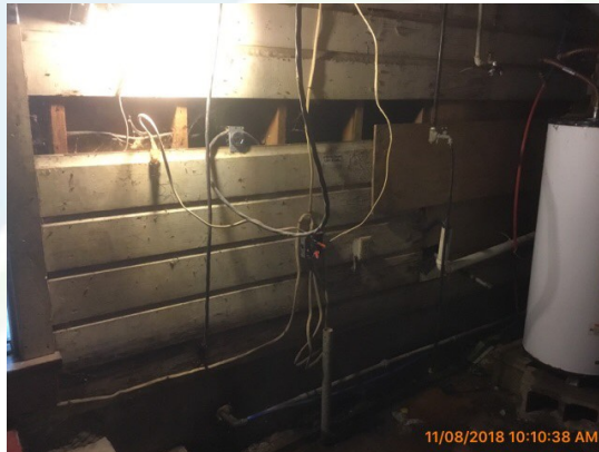
East garage wall
